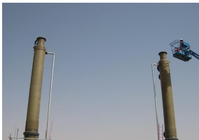
Figure 1 SO 2 absorption towers
