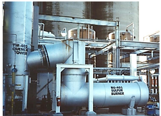
Figure 3 CellChem Spiral Flame Furnace
